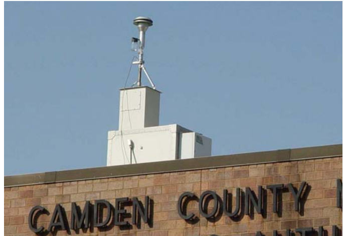
Figure 1: Ambient air monitoring sampler located on the roof of the Camden County Municipal Utilities Authority Building
